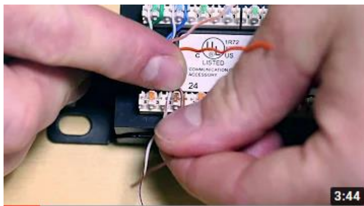
Figure 21 - Video about mounting a copper patch panel
