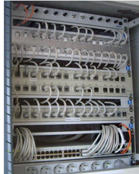
Figure 2 - Telecommunications enclosure
